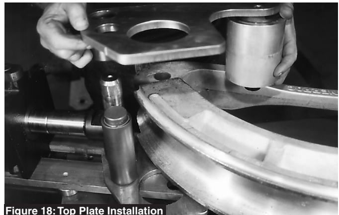
Figure 18: Top Plate Installation
