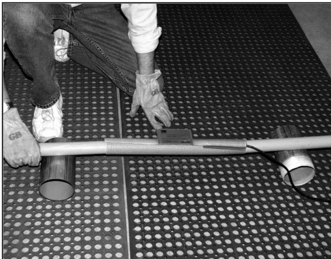
3. Plug power cord in a 120V AC outlet. Wait 4 or 5 minutes, then check pipe flexibility by trying to bend it. If pipe resists bending, leave blanket on for 2 or 3 minutes longer. When the pipe bends easily, remove and unplug the blanket.
